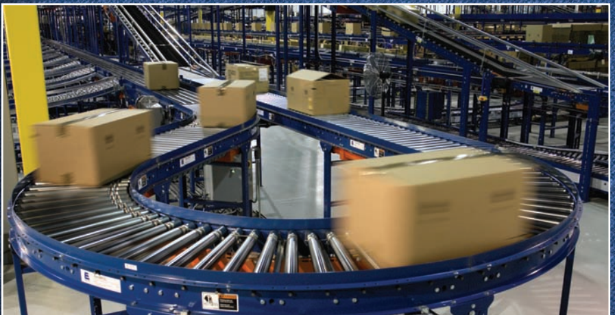
Real-time interfaces between the WMS and WCS directs the scanned outbound carton to either go to value-added services for additional operations requested by customers, to an outbound quality check, or to an automated print-and-apply area for shipment.
