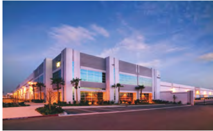
The ProLogis Kaiser Commerce Center, which comprises approximately 5.9 million square feet in nine buildings, is now fully occupied with a recent lease agreement of 484,000 square feet to a leading 3PL.
