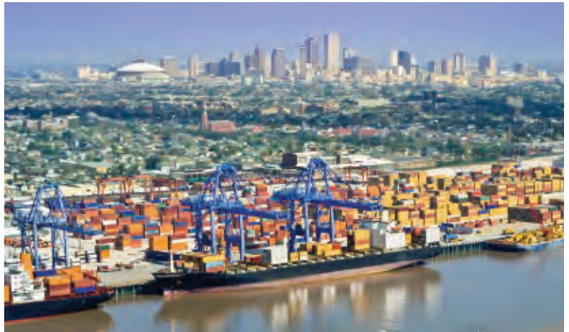
Enhanced intermodal projects are underway in the Gulf port of New Orleans thanks to the U.S. DOT’s popular TIGER grants program.
