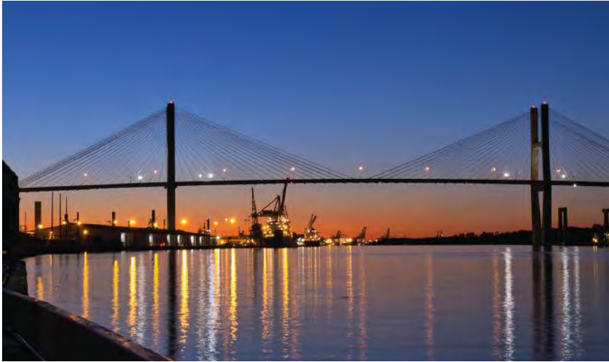
Deepening the Savannah Harbor from 42 feet to 47 feet will accommodate an increase in the number of super-sized container vessels transiting the Panama Canal after its 2015 expansion.
